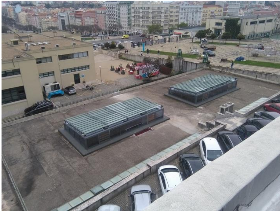
Figure 5.3 - Roof of Pavilhão de Informática II
